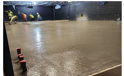
Above: Stage slab being placed.
